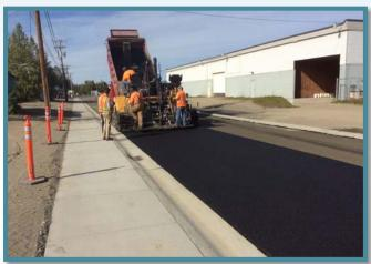
North Aspen Drive Improvements – The existing street was a gravel road in poor condition with inadequate drainage and required considerable maintenance. The project reconstructed the subgrade, replaced an aging AC water main and paved the street with curb, gutter, sidewalk on one side and street lighting. The approximately 900 foot long street remains one of the few commercial streets in Soldotna that has available land for development.
